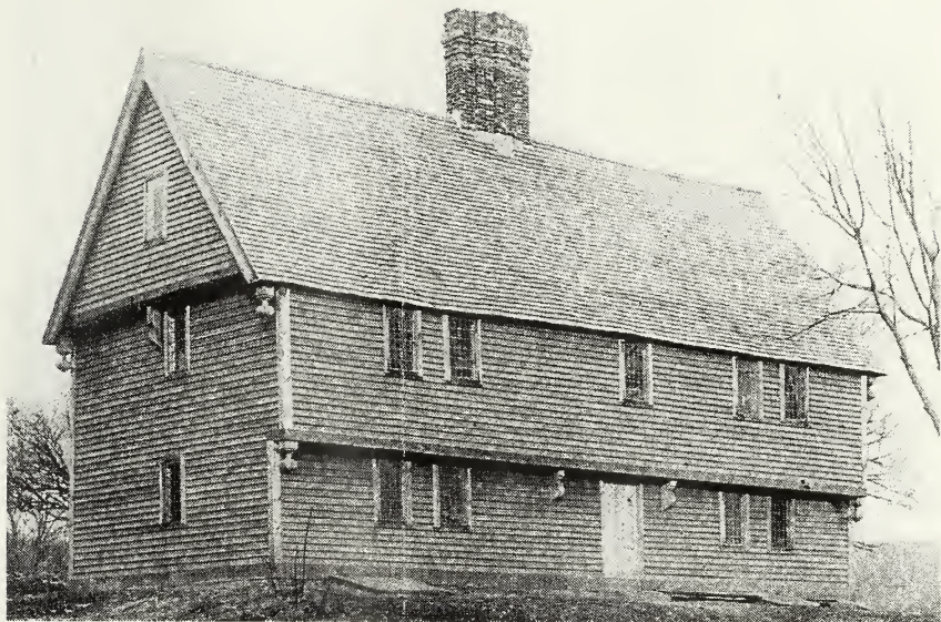
The Capen House shortly after the restoration. The clapboards and trim were left to weather naturally, and did not receive any opaque finishes until the current treatment of dark brown stain was initiated in the 1970s.
